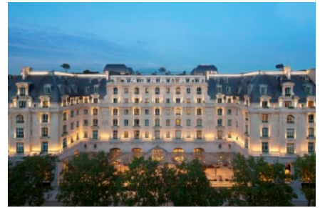
Hotel Peninsula Câble chauffant
