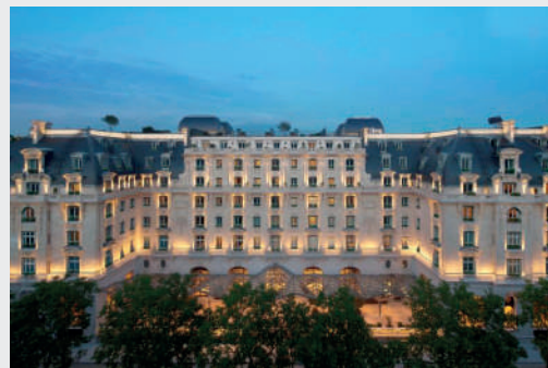
Hotel Peninsula Câble chauffant
