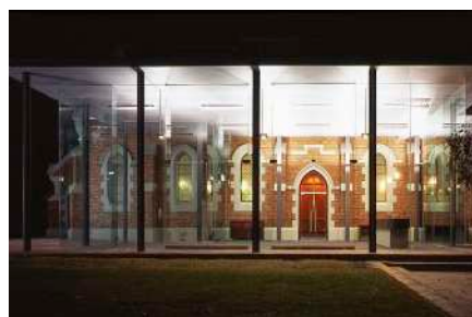
St. Michaels Church , Australie Panneaux rayonnants
