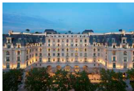
Hotel Peninsula Câble chauffant
